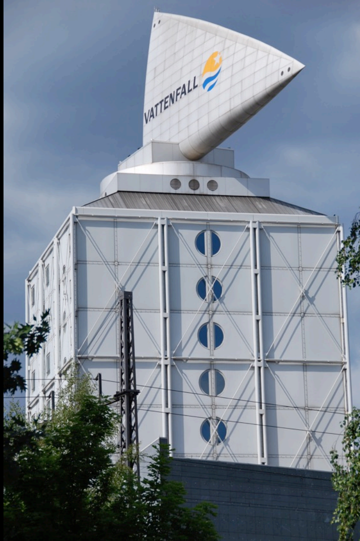
Kant-Dreieck Office Building Berlin, Germany Josef Paul Kleihues
